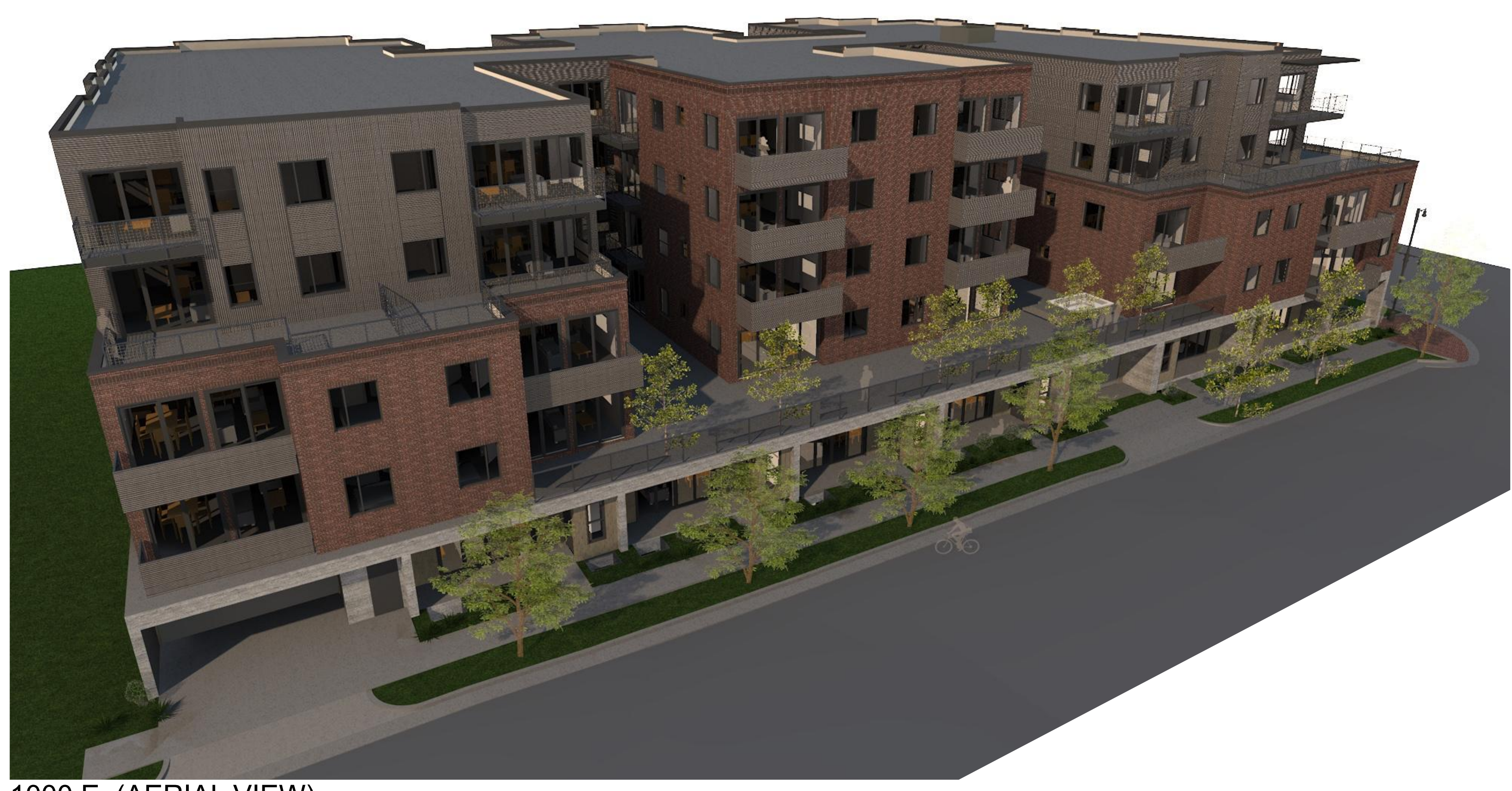
1000 E. (AERIAL VIEW)
